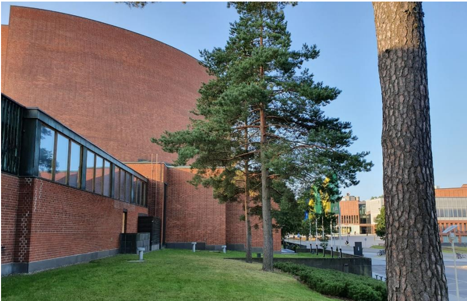
Figure 1: The Aalto campus, with the Candidate Centre building in the front of the picture.
