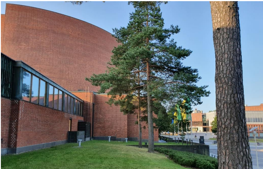
Figure 1: The Aalto campus, with the Candidate Centre building in the front of the picture.
