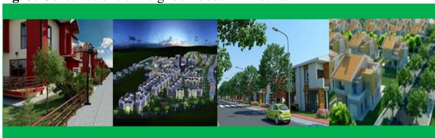
Fig. 3: Constructions of neighborhoods in Pristina.
