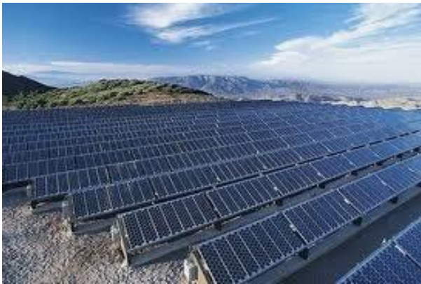
Fig.3. Display of a photovoltaic solar farm
