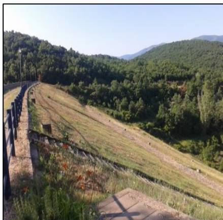
Fig.2. Downstream side of dam
