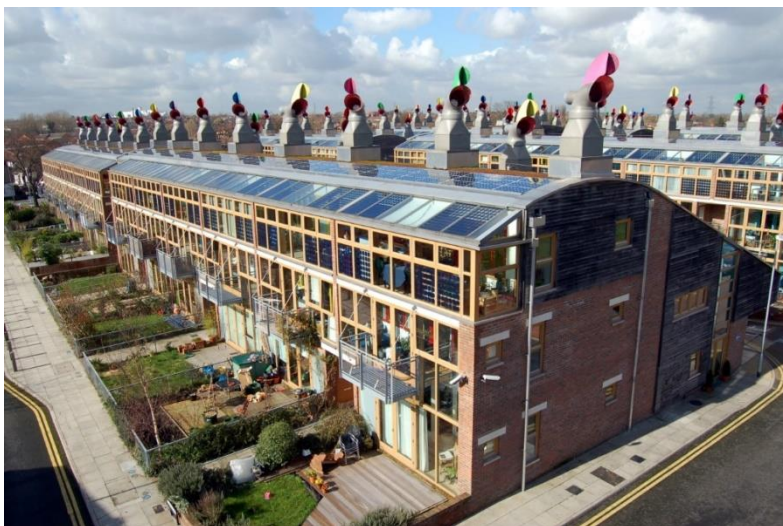
Photo: Beddington Zero Energy Development (BedZED) London, Tom Chance from Peckham, 2007 Reproduced by Permission.
