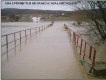
Figure 1: Floods in Drenica river, 2006
